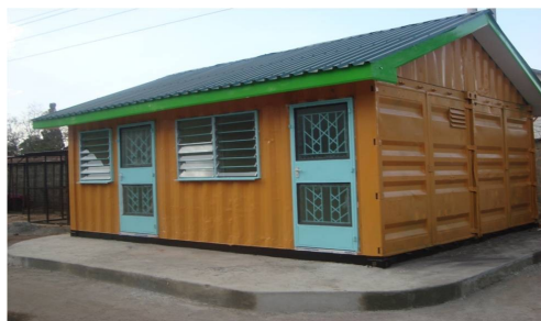
Nairobi office and reception renovations
